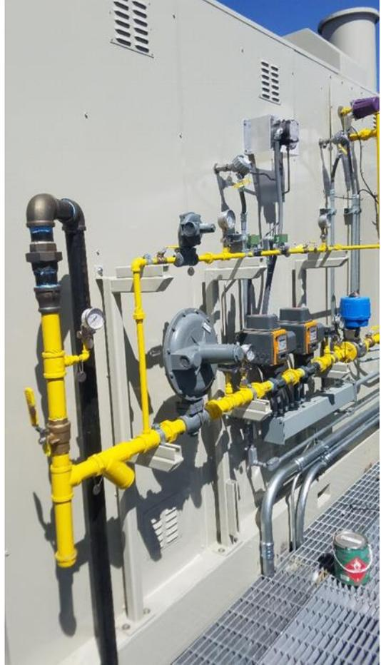
*Side Views of the Catalytic Oxidizer NFPA Gas Train*
