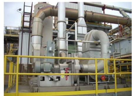
*Right: The Pollution Systems VS-3 Venturi Scrubber System installed at a pork sausage plant in Alabama*
