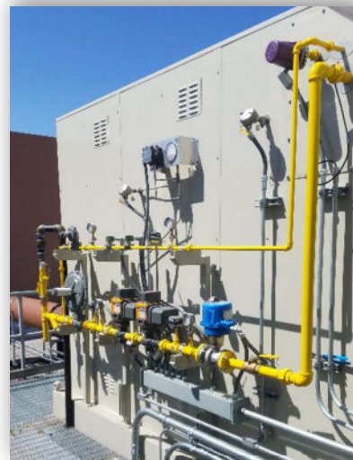
Side Views of the Catalytic Oxidizer NFA Gas Train
