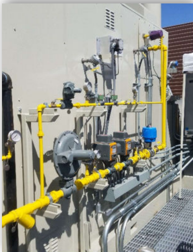
Side Views of the Catalytic Oxidizer NFA Gas Train
